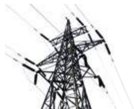
ENERGY TRANSMISSION TOWER
