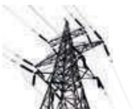
ENERGY TRANSMISSION TOWER
