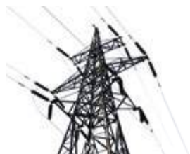
ENERGY TRANSMISSION TOWER
