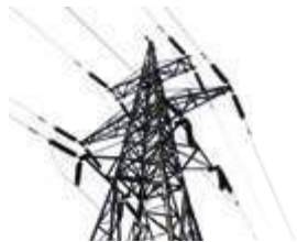
ENERGY TRANSMISSION TOWER
