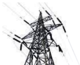
ENERGY TRANSMISSION TOWER
